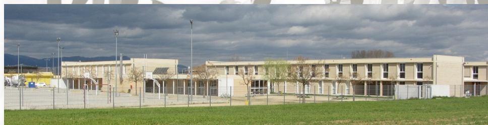
Institut Vidreres i zones del voltant.
